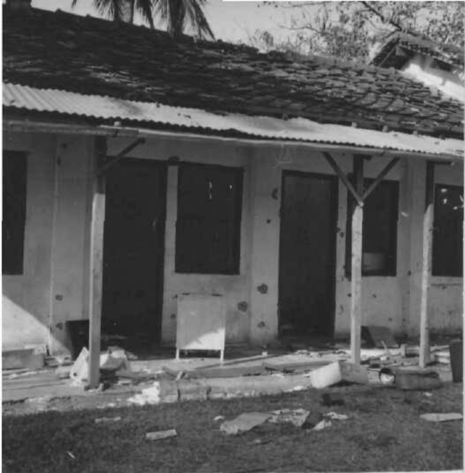
SERVANTS' QUARTERS MISSIONARIES SOUGHT REFUGE HERE BEFORE ENTERING BUNKER 19.38-16
